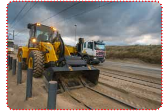
Sand can pile up over a considerable distance by as much as half a yard in height.
